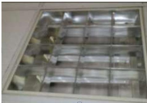
**Figure 5:** Fluorescent tube lighting fitting 72W 2 feet x 2ft (Saleh, 2017)
