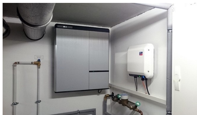
Figure 12: LG Chem’s RESU installed for residential power (Casey, 2019)
