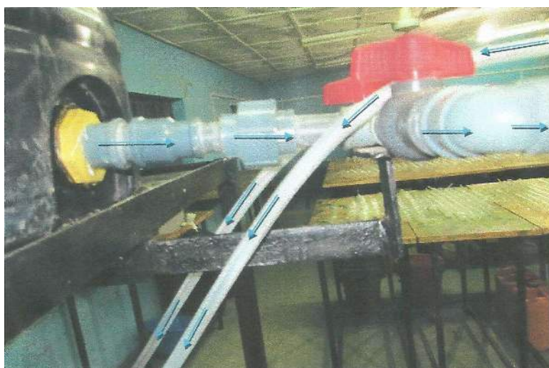
Plate II: Arrows Showing the Directions of Coolant Flow
